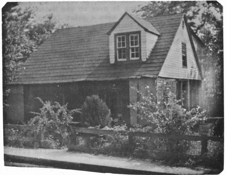
30 Wellesley Circle in the throes of rehabilitation.
