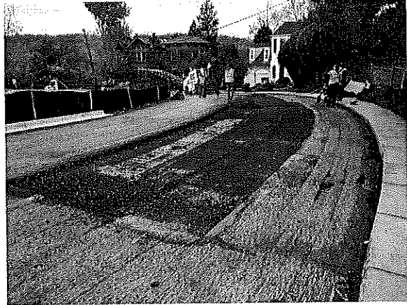
Inadequate base milled away.
