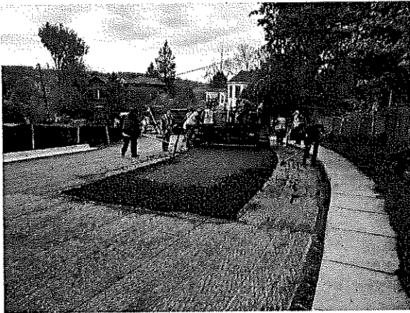
Base repair paving underway.
