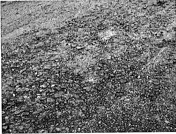
Loose stone and rubble of inadequate base.
