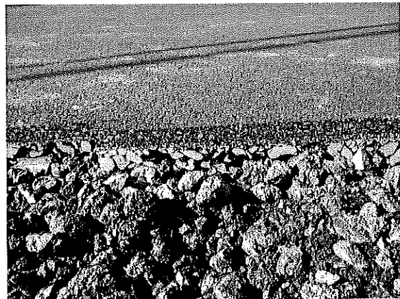
A cross-section of an inadequate base.
