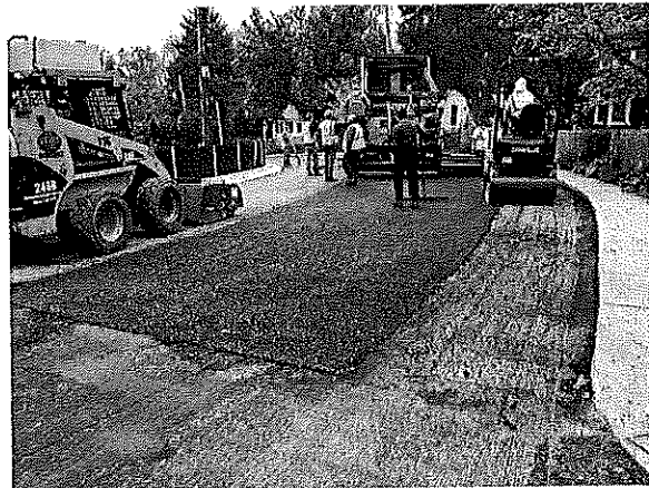
Base paving rolled out.
