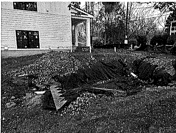
The partially completed landscape infiltration facility.
