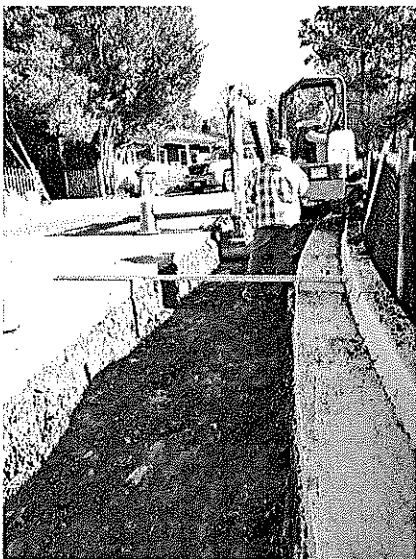
Excavation underway to a suitable base, and filled with compacted gravel for the pavement base.
