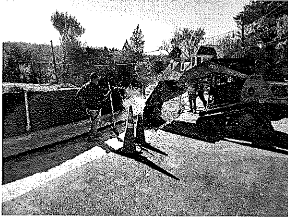
Asphalt placement and compaction.
