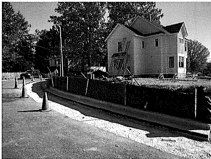
Excavation underway to a suitable base, and filled with compacted gravel for the pavement base.
