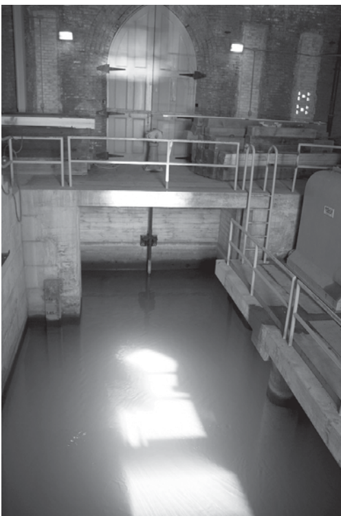
Georgetown Reservoir pumping station: its exterior above and its interior (inset photo), showing the pool of water where the eels swim
