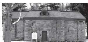
The Gatehouse (no longer used) at Great Falls
